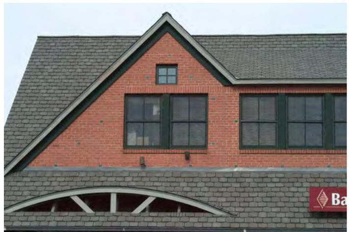
AN EFFECTIVE EXAMPLE OF SHADOW LINES & COLORING IN A MODERATELY PRICED LAMINATED SHINGLE
