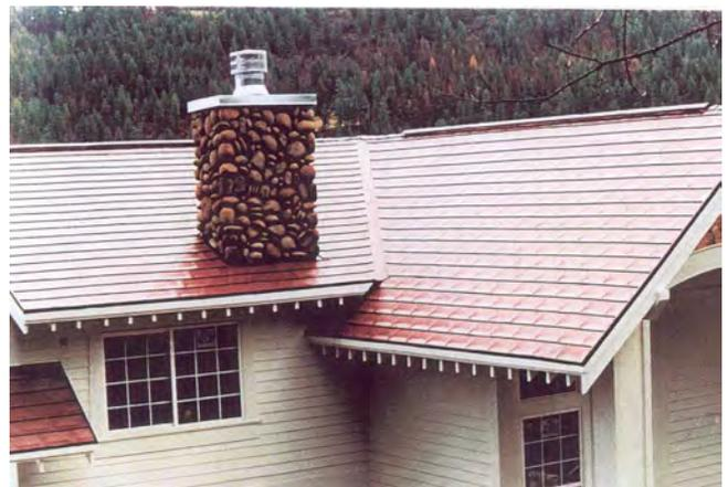
THE TWO MAIN OBJECTIONS TO PAINTED METAL ROOFING IN STARWOOD HAVE BEEN THE REFLECTIVITY AND THE STRONG COLORING / PIGMENTATION
