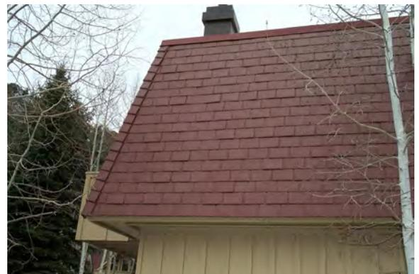
A LESS SUCCESSFUL INSTALLATION OF ECOSTAR SYNTHETIC SLATE TILES - SLOPE IS TOO VERTICAL FOR THESE TILES AND COLOR ACCENTUATES MONOCHROMATIC “MANUFACTURED” QUALITY
